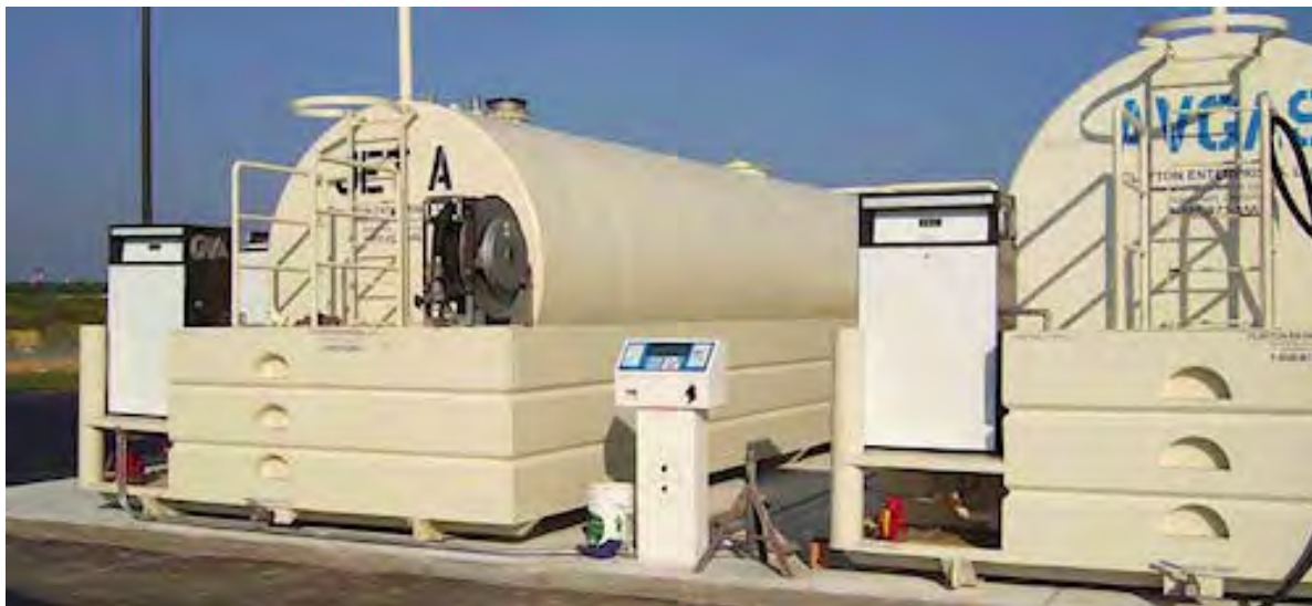
Figure 22: This illustrates a typical "self-serve" refueling system. It has two tanks, one for Jet-A and one for 100LL. It processes payments using a credit card reader.
