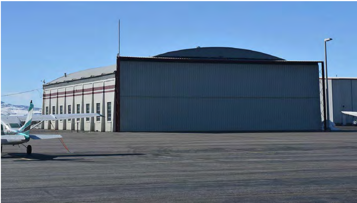
Figure 10: One of the larger hangars on the field is this handsome building, a remnant of the Second World War. It houses corporate aircraft used by a Logan company which has customers across the entire U.S.
